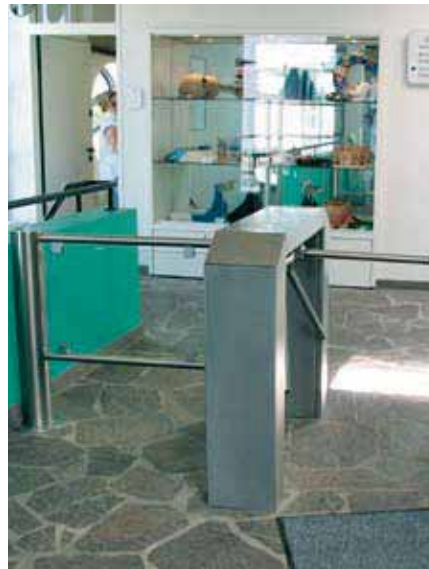
An automatic swing door beside the tripod barrier provides access for people with reduced mobility
